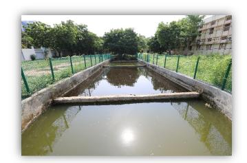
The land surface behind the L - building have been sloped toward the rainwater collecting pond in order to collect all the rain water that drains from the surrounding areas. Safety fencing and paver block pathway were provided around the pond.
